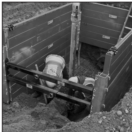
Three-sided configuration with telescoping spreaders and removed bottom panel
