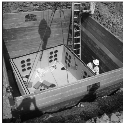
Long paneled four-sided configuration with sectional corner posts
